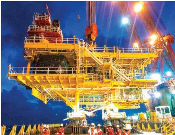
Photo shows offshore wellhead platform installation work during Phase 2 of the bundled natural gas development project in the Gulf of Thailand. PHOTO: NIPPON STEEL ENGINEERING CO./NNA/KYODO
