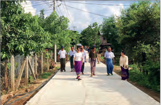
Officials oversee the progress of the concrete road construction project in Tatkon Township.
