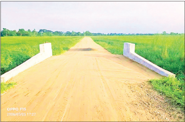
This image captures the completed status of the pipe culvert structure along the rural product transport road in Dekkhinathiri Township.
