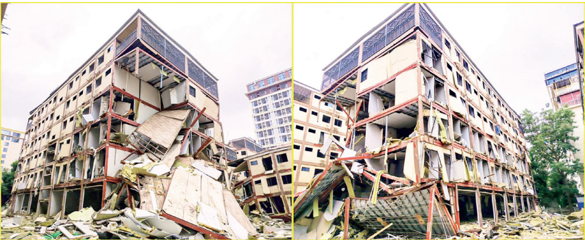
An illicit scam-related seven-storey structure is seen following the demolition.
