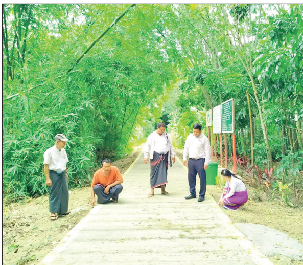
Officials oversee the ongoing village concrete road construction in Maubin Township, Ayeyawady Region.
