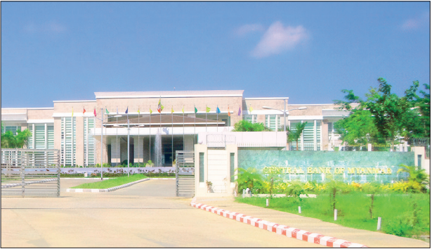
A facade of the Central Bank of Myanmar (CBM) in Nay Pyi Taw.
