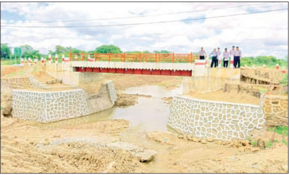
Officials inspect the completed concrete bridge in Minbu (Sagu) Township.
