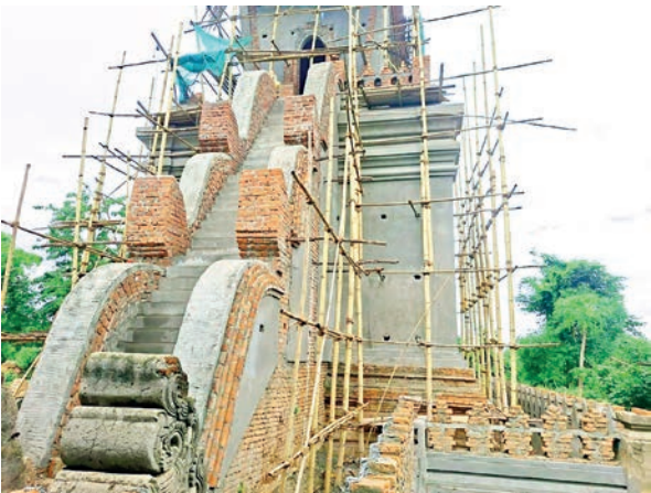
A view of the Inwa tooth relic building reconstruction.
