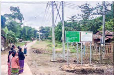
Officials inspect the completed installation of the 400V power line in Pantanaw Township.
